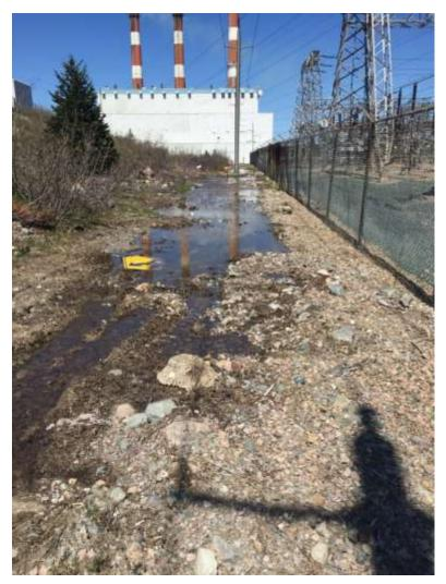
Figure 2: Flooding Near the Terminal Station due to a Break on the Tank Farm Firewater Loop
