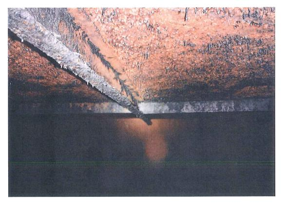
Minor twist in rafter monitor at next Internal Inspection
