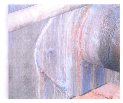
Nozzle Repad plugged and this should be removed and replaced with silicone
