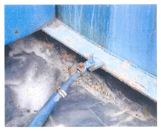
Grounding cable attached and in good condition
