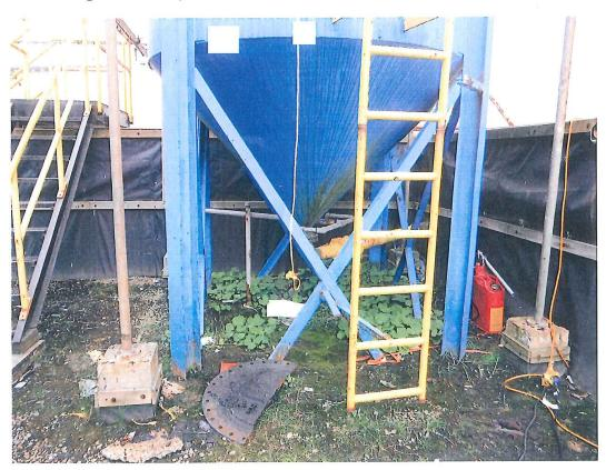
Structural legs buried and covered with moss and vegetation no evidence of Liner under the legs of the additive tank
