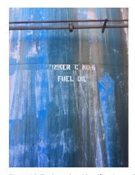
Figure 16: Tank product identification and staining on shell from corrosion on roof.
