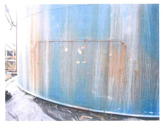
Leak area, chine undermining, and exposed liner
