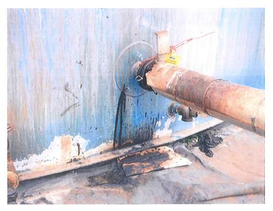
Tank chine area undermined and exposed dyke liner repad plugged recommend removal and replace with silicone
