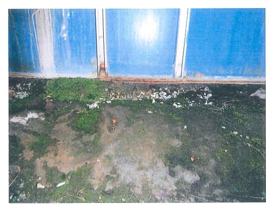
Vegetation and exposed liner around tank pedestal and base of tank.
