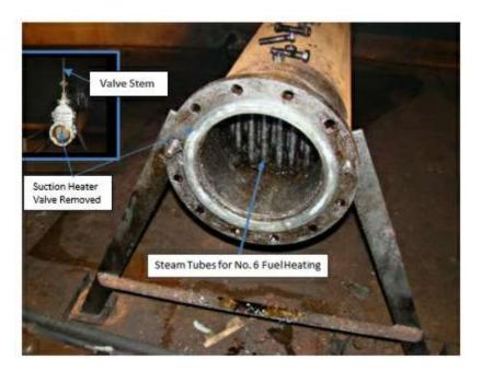
Figure 2: Tank 2 Suction Heater
