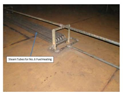
Figure 3: Tank 2 Platform Heater
