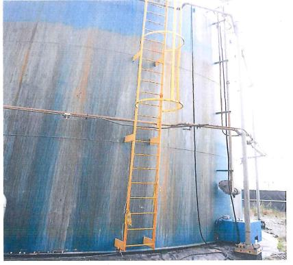
Ladder in Good condition exposed liner evident
